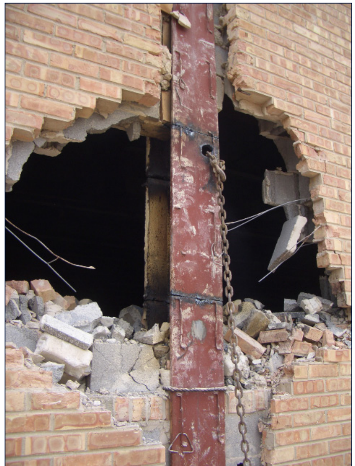
Figure 9. Torched Column Ready to be Pulled Out.
