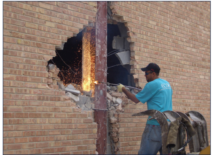
Figure 8. Column 16C Being Torched.
