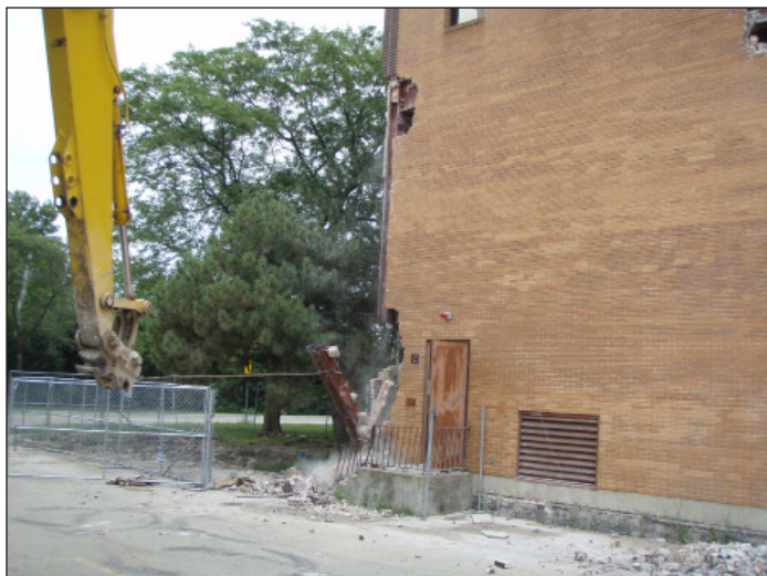
Figure 10. Torched Section of Column 11C Being Removed.
